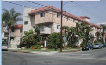
NEBRASKA AVE., WEST LA, CA -- 26 UNITS
