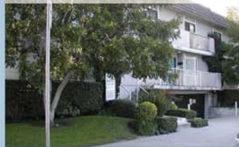
WHITSETT AVE., VALLEY VILLAGE, CA -- 21 UNITS
